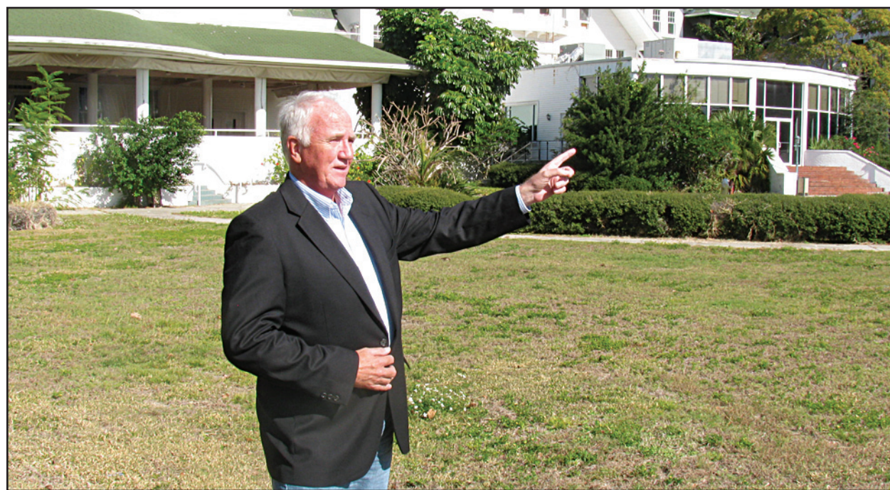
Photo by BRIAN GOFF Matt Cummings, managing member of the Belleview Biltmore ownership group, stands in front of the historic, deteriorating hotel. The owners plan to ask for a demolition permit in January.
